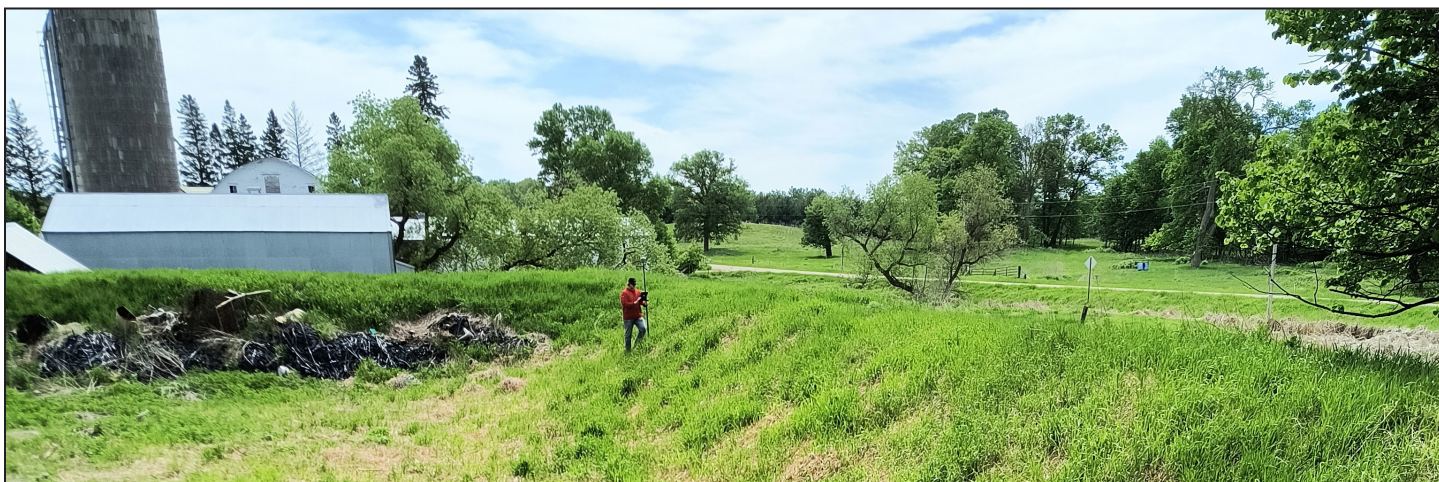
Ethan Bachmann, a Becker SWCD engineering technician working on behalf of TSA 1, surveyed the site of an unused agricultural waste facility in Otter Tail County in June. The site is being prepared for closure as part of a project identified as a priority in the Otter Tail River Comprehensive Watershed Management Plan developed via BWSR's One Watershed, One Plan program. Photo Credit: Becker SWCD
