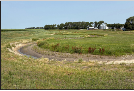
Left: Most of the 4-mile-long upstream segment of the Swift Coulee restoration was dry in mid-July. Before, the 4-inch rainfall total for June would have destroyed crops in parts of adjacent fields. Middle: Side-water inlets let water slowly meter off the landscape. When the coulee spills into the constructed floodplain, flap gates keep floodwater from backing up onto adjacent property. Right: A tile line was relocated as part of the project. Here, a field borders a levy and floodplain.
