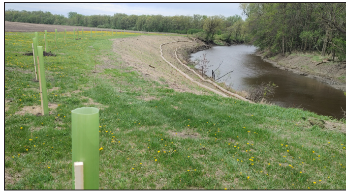
Top: One of the district's primary activities for its One Watershed, One Plan work is stabilizing eroding streambanks in the Red Lake River, Clearwater River and Thief River. Toe-wood sod mat stabilization was installed along the Thief River in 2024, with vegetation established the following year. Bottom: Local agencies and artistic volunteers completed storm drain stenciling as part of a stormwater treatment project designed to help protect drinking water for the City of Thief River Falls. The project was substantially completed in 2025.
