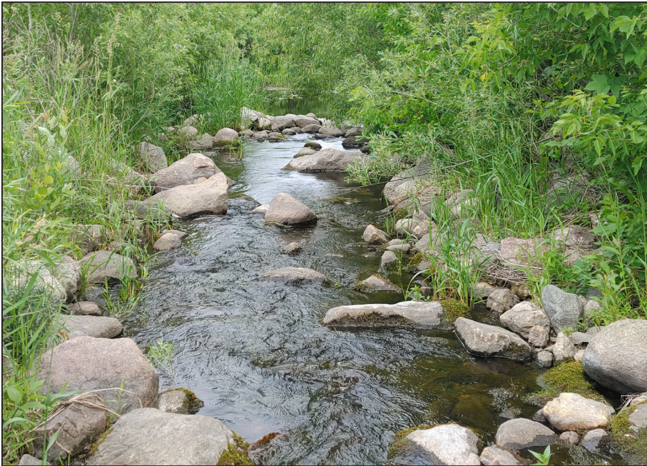
Left: The Spring Gravel Dam project in Polk County at the headwaters of Burnham Creek is one example of projects the Red Lake Watershed District pursues to meet local water quality goals. The project installed rock riffles to stabilize the streambank after a washout. Top right: District staff members (from left) Lindsey Deselich, Corey Hanson, Tony Olson, Erick Huseuth, Tammy Audette, Melissa Bushy, Nate Koland and Elaine Rychlock were among the people surveyed as part of the PRAP assessment process. Bottom right: District board members (clockwise from top left) Tom Anderson, LeRoy Ose, Grant Nelson, Allan Page, Terry Sorenson, Gene Tiedemann and Brian Dwight also participated in the survey process.
