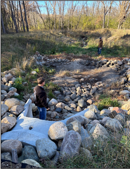
Left: Brainerd Public Works Director Mike Habighorst, left, and BWSR Board Conservationist Darren Mayers, who is now BWSR's easement programs and forestry coordinator, explored a rock-armed plunge pool on Oct. 23, 2025, in Brainerd. The pool filters stormwater runoff bound for Little Buffalo Creek. Middle: From left: Habighorst, Mayers, Crow Wing SWCD Manager Melissa Barrick and Brainerd City Engineer Jessie Dehn paused at one of 22 manholes, which were installed at every bend of a 1,300-foot-long pipe that runs the length of the gully. Right: Erosion control logs help to stabilize the gully, which developed as the result of channelized flow created by a culvert installed under a road in the 1980s. Photo Credits: Ann Wessel, BWSR
