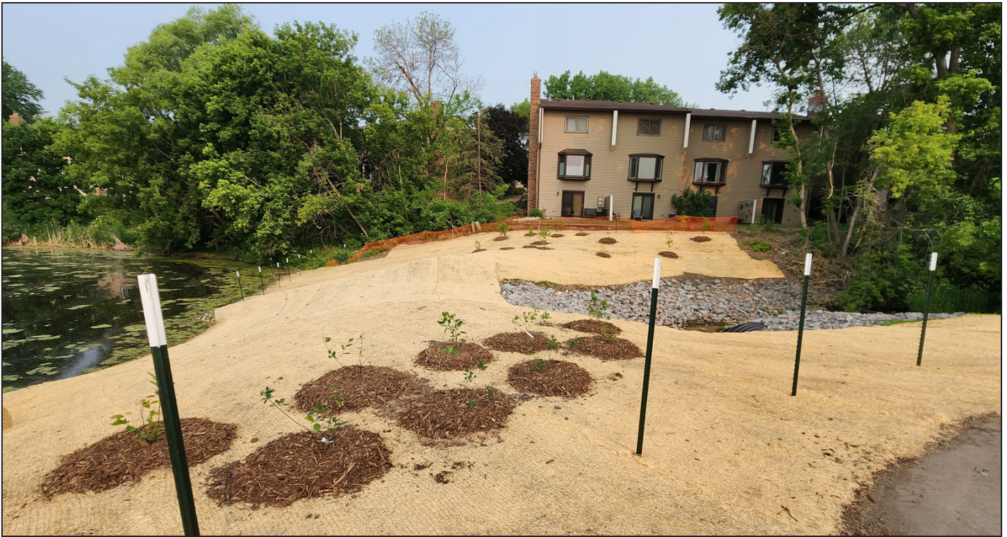
Native vegetation was established throughout the project area to provide enhanced habitat and improved water quality. Shorelines that are stabilized with native plants are less susceptible to bank erosion. Native plants' deep root systems also play a key role in water filtration by absorbing pollutants and excess nutrients.
