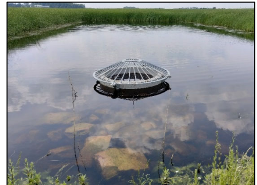
An inlet feeds water to a structure containing an internal weir that helps control water levels in a restored wetland.
