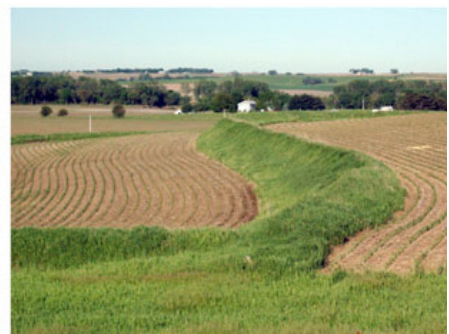
Left to right: A water and sediment control basin in crop field is empty in dry conditions but holds water temporarily after heavy rains; landowners pose by construction of storage basin in a Pope County ag field; grass back sediment control basin slows runoff. Photo Credits: BWSR
