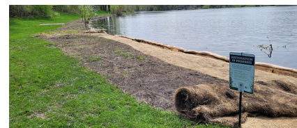
A prepared seedbed where erosion fabric is being applied after seeding
