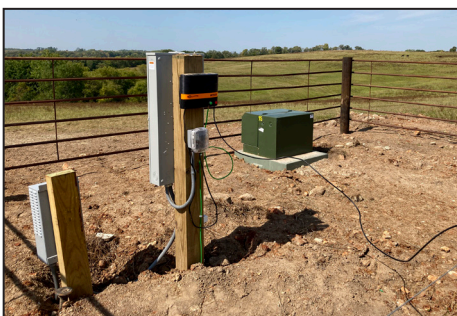
An electricity-powered pumping station, left , a 568-foot-deep well and pipes that carry water to tanks are among the elements that made rotational grazing possible on 70 acres in Fillmore County, middle . Enclosing the pasture and dividing the paddocks took nearly 3 miles of high-tensile fencing.
