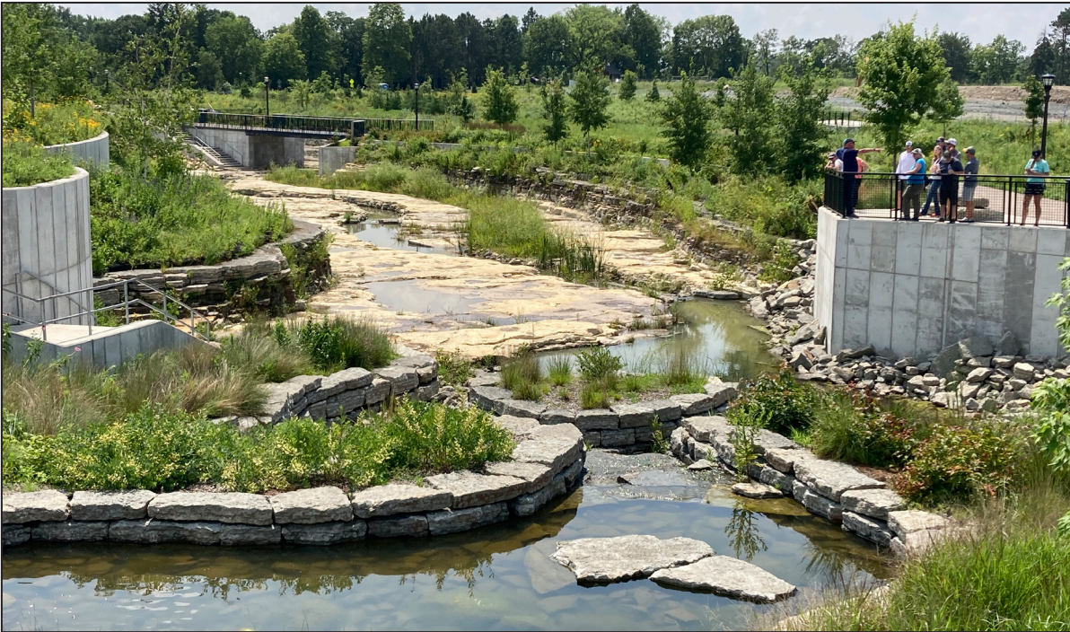
Tour attendees viewed Hidden Falls Creek at Highland Bridge. Located upstream, the central water feature can collect and clean up to 64 million gallons of stormwater annually from the 122-acre site of the former Ford manufacturing plant. Photo Credits: Anne Sawyer, BWSR
