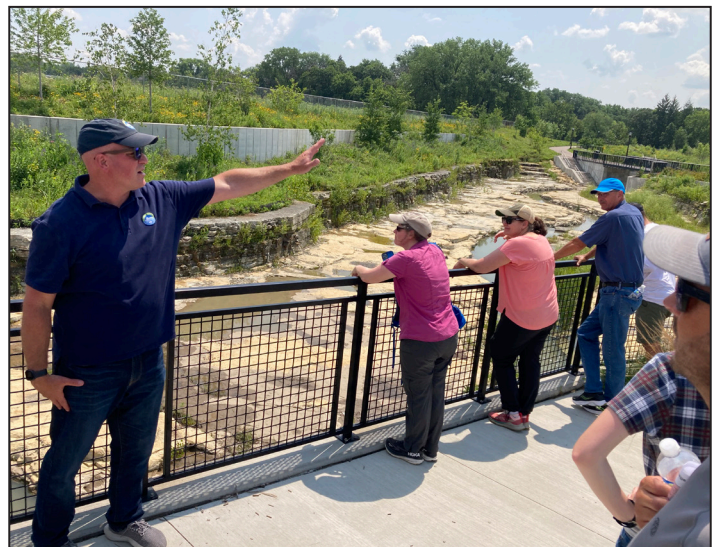
Capitol Region Watershed District Deputy Administrator Bob Fossum discussed site redevelopment at the Highland Bridge site in St. Paul, including Hidden Falls Creek, which once flowed through an underground storm sewer pipe. Today, a segment of the creek flows through a channel in existing bedrock, making its way toward Hidden Falls Regional Park and the Mississippi River. The creek is surrounded by rain gardens and native plants that collect and filter overland stormwater flow while providing pollinator habitat and landscaping.
