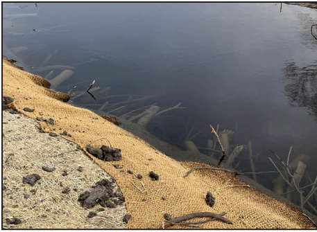
Left: Toe wood, submerged logs anchored into the streambank, seen here in March 2024, helps to stabilize the banks and slow the flow of water in the restored segment of the South Fork Rush Creek. Center: A city trail project, which is adjacent to but not funded by the WBIF stream restoration, will become part of Three Rivers Park District’s regional trails system. The path leads to a new steel-truss bridge that spans the restored segment of the creek. Right: Water flowed over a constructed riffle in March 2024 in a segment of the restored creek.
