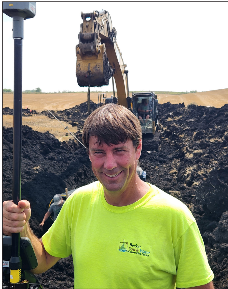
Becker SWCD-based South Pod Engineer Wes Drake staked tile lines and conducted post-installation surveys in August within the West Otter Tail County district where construction of a stabilization structure and water and sediment control basins was underway. Photo courtesy of Wes Drake
