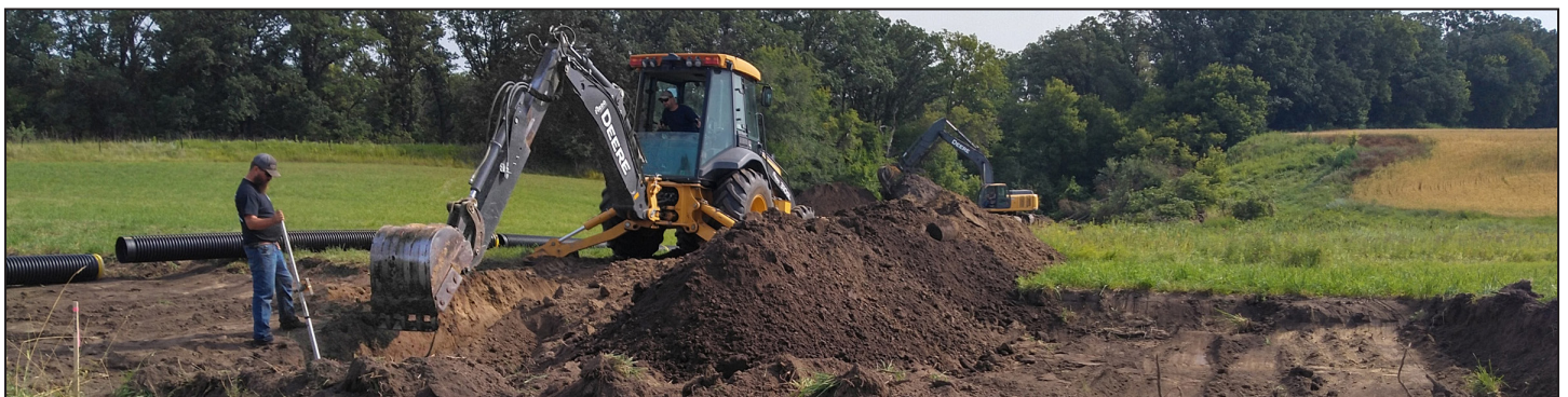
Projects involving North Pod engineering staff included a grade stabilization in Red Lake County. Photo courtesy of Red Lake County SWCD
