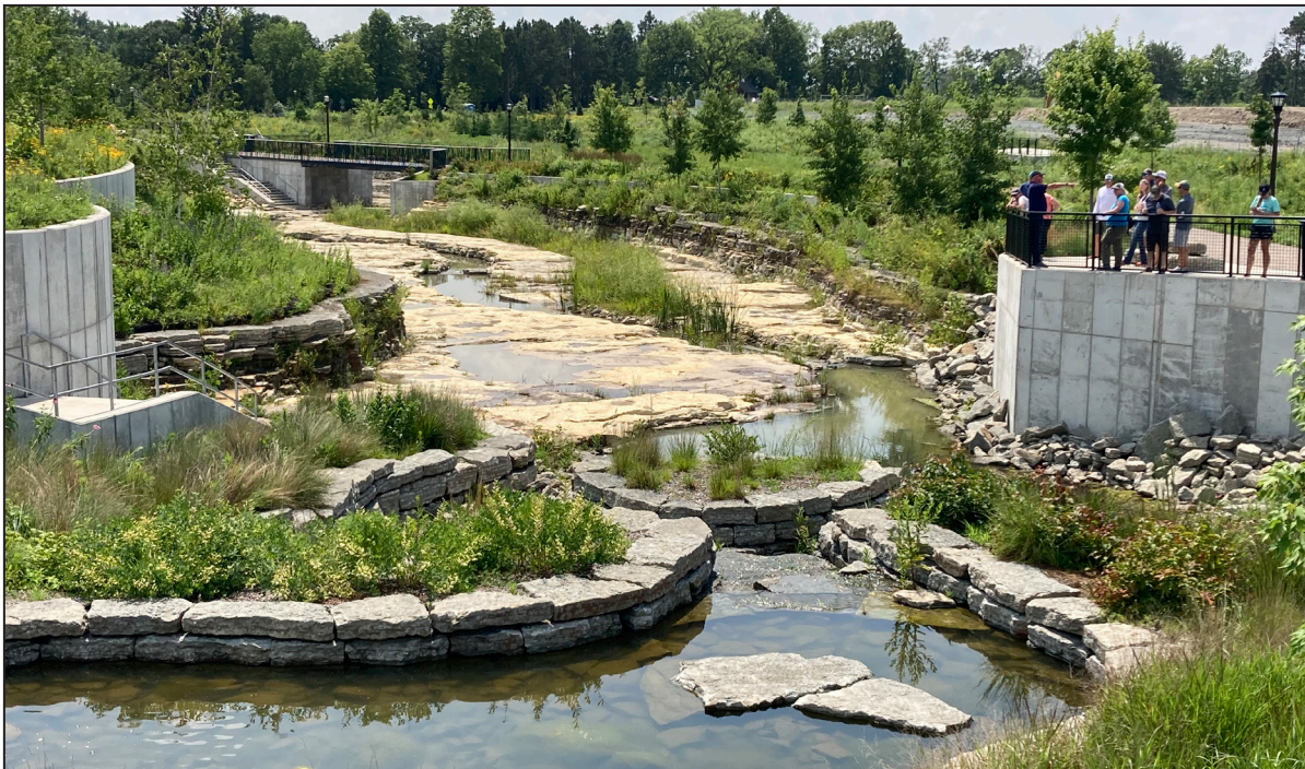
Tour attendees viewed Hidden Falls Creek at Highland Bridge. Located upstream, the central water feature can collect and clean up to 64 million gallons of stormwater annually from the 122-acre site of the former Ford manufacturing plant. Photo Credits: Anne Sawyer, BWSR
