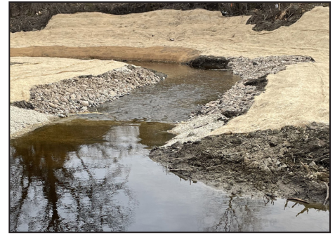
Left: Toe wood, submerged logs anchored into the streambank, seen here in March 2024, helps to stabilize the banks and slow the flow of water in the restored segment of the South Fork Rush Creek. Center: A city trail project, which is adjacent to but not funded by the WBIF stream restoration, will become part of Three Rivers Park District’s regional trails system. The path leads to a new steel-truss bridge that spans the restored segment of the creek. Right: Water flowed over a constructed riffle in March 2024 in a segment of the restored creek.
