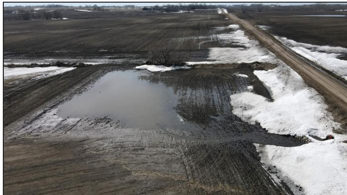
After a sudden warmup followed heavy snows, a water and sediment control basin worked as designed in spring 2023 in a field Mark Thompson farms in the East Branch Chippewa River watershed. Before the basin was installed, a sudden spring melt would have carved gullies into the field. **Photo Credit:** Andy Albertsen, Swift County SWCD
