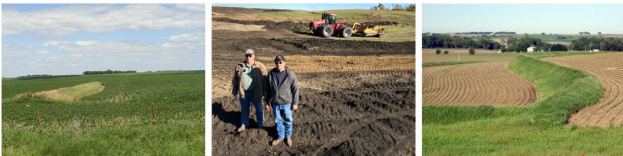
Left to right: A water and sediment control basin in crop field is empty in dry conditions but holds water temporarily after heavy rains; landowners pose by construction of storage basin in a Pope County ag field; grass back sediment control basin slows runoff.
