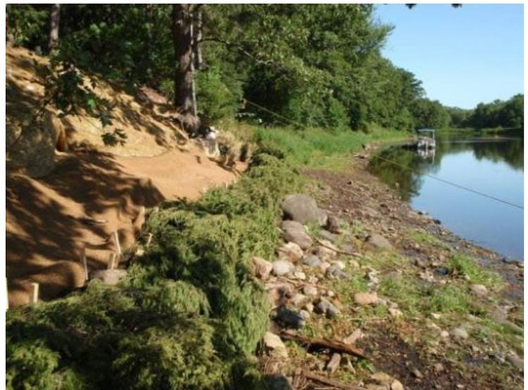
Bank stabilization with cedar revetments and erosion control blanket along the St. Croix River
