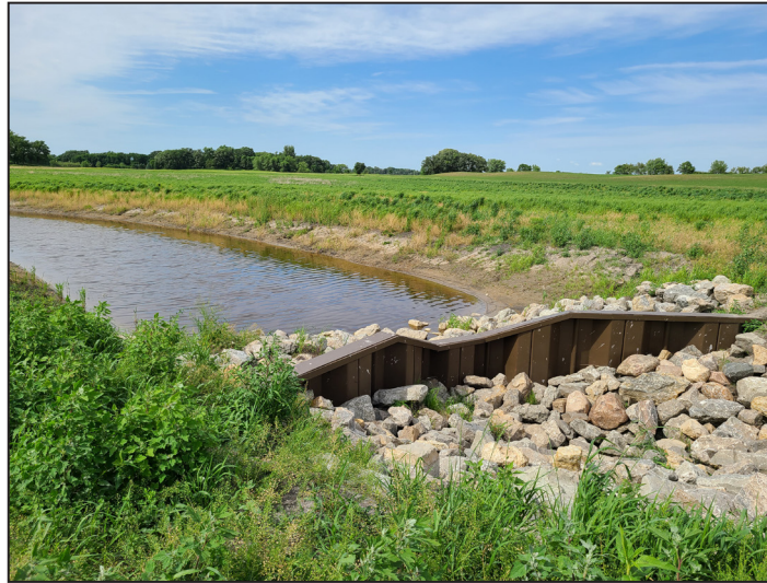
Above: An outlet structure installed on a Freeborn County MN CREP easement provides water storage. Photo Credit: Freeborn SWCD
