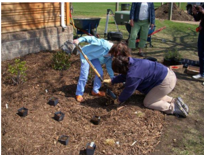
Raingarden where mulch has been applied before planting to prevent compaction
