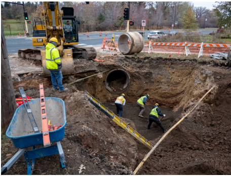
Work started in October 2020. Construction was coordinated with planned street improvements to save money and minimize traffic disruptions in the neighborhood. Restoration and planting followed storm sewer replacement and grading.
