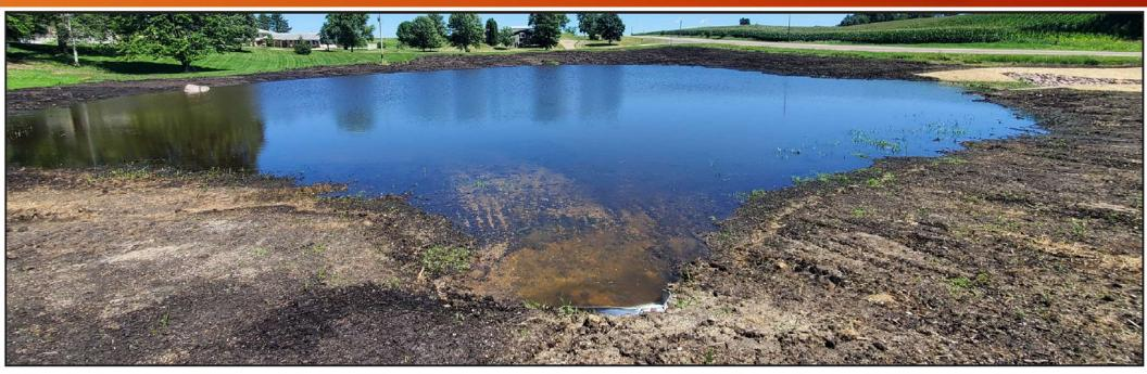
Contractors in summer 2020 excavated more of the wetland to increase flood storage, and installed a culvert connecting it to the upper watershed. **Photo Credit:** Le Sueur County SWCD
