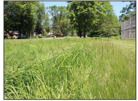
A spent lime filter on the north side of Silver Lake, left, diverts stormwater to a basin and then to a wetland, treating the water before it enters the lake, removing dissolved phosphorus by binding it to calcium carbonate. On the south side of the lake, a restored bio-retention basin, middle and right, allows nutrients and the pollutants they carry to settle out. Photo Credits: Greg Williams, Barr Engineering
