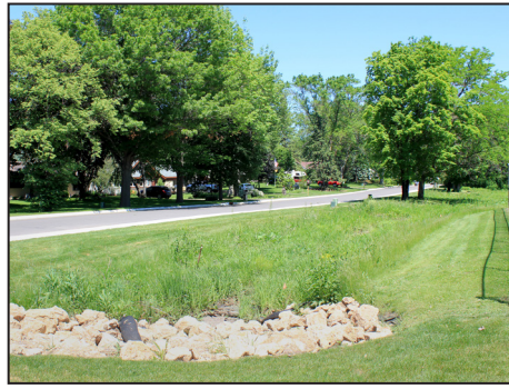
A spent lime filter on the north side of Silver Lake, left, diverts stormwater to a basin and then to a wetland, treating the water before it enters the lake, removing dissolved phosphorus by binding it to calcium carbonate. On the south side of the lake, a restored bio-retention basin, middle and right, allows nutrients and the pollutants they carry to settle out. Photo Credits: Greg Williams, Barr Engineering
