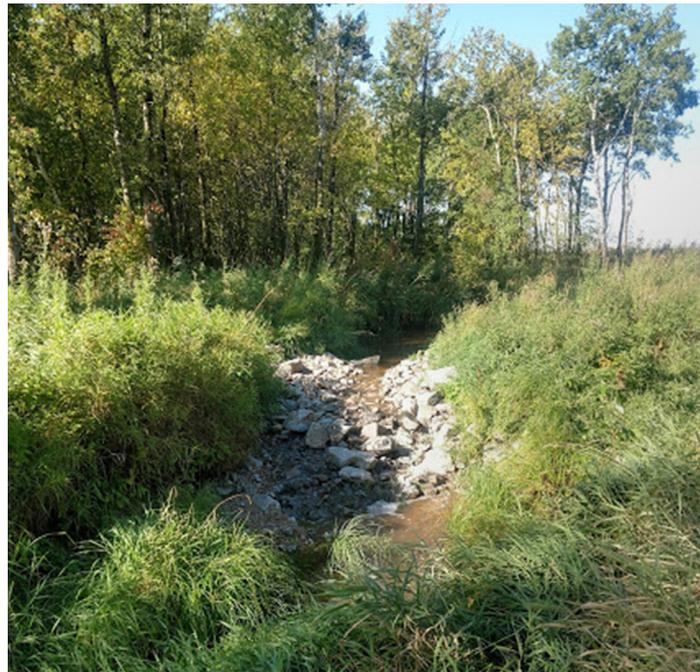
*The vegetated drop structure, the only element of the County Ditch 8 project damaged since construction, is pictured here one month after repairs. Photo Credit: Torin McCormack, RRWD*
