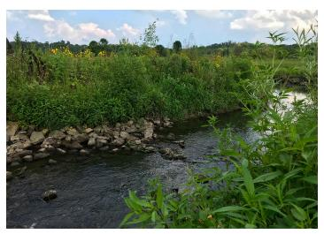
**Top:** The redesigned South Branch of Cascade Creek mimicked the sinuosity, dimension and shape of a stable channel elsewhere in the watershed. **Bottom:** Wetlands eventually will fill with water. Logs and roots will help to create habitat.
