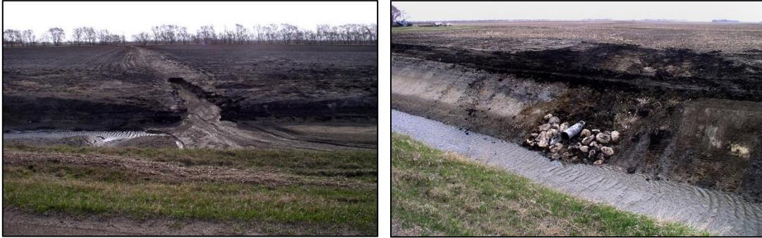
*Left: Previously, uncontrolled runoff caused severe erosion that contributed to Otter Tail River pollution. Right: Now, side-inlet structures control field runoff, reduce erosion and improve water quality in the Otter Tail River.*
