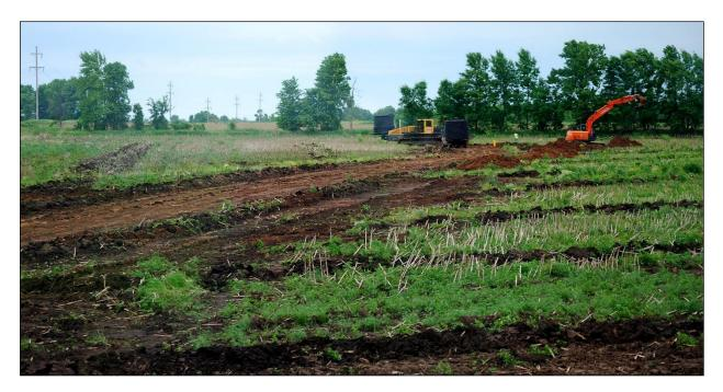
Work on Czech's 23-acre field included construction of a water and sediment control basin, using Clean Water Fund dollars. It was built in conjunction with a tiling project that Czech paid for himself.
