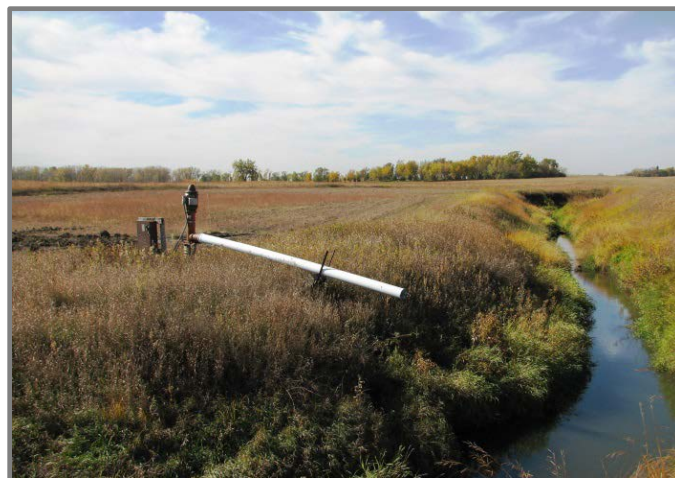
Figure 1. Tile Drained Wetland Aided by Lift Station
