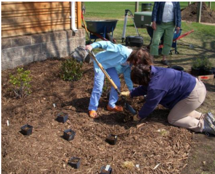
Raingarden where mulch has been applied before planting to prevent compaction Photo: Metro Blooms
