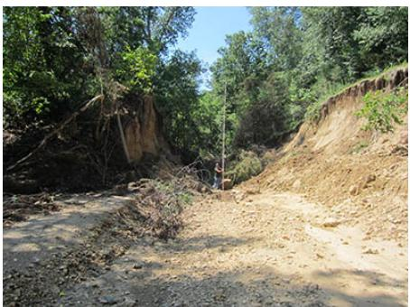
One of the major projects was an earthen dam that blew out during the heavy rainfalls, sending approximately 5,500 tons of sediment downstream and leaving unstable vertical banks behind. Constructed in the 1970s, to provide rate control for an upland watershed to the Cannon River, there was not enough funding available to replace the dam. Those banks were a safety risk in the park, though, which made repairs on the public land eligible for FEMA funding.
