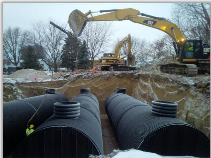
*Phase two of the project installed three storage tanks that will be used to hold water.*
