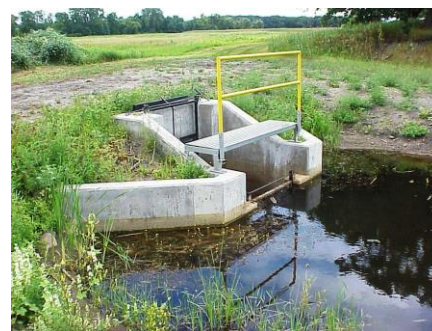
Wetland outlet that can be used to control water levels
