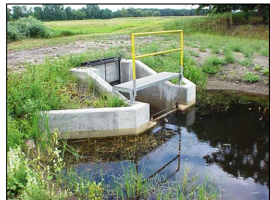
Wetland outlet that can be used to control water levels
