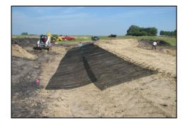
of the embankment front slope. More detailed discussion of these strategies for preventing muskrat damage to constructed embankments occurs in Section 4-4, Engineering Design and Construction, Earthen Embankments - Other Design Considerations.
