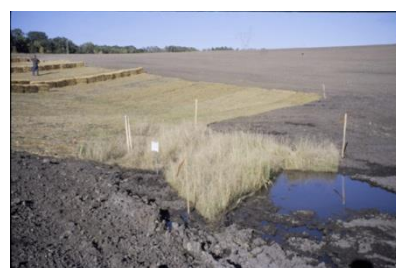
Prevegetated mats, erosion fabric and straw bales stabilizing a swale
