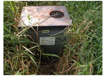
Water level control
