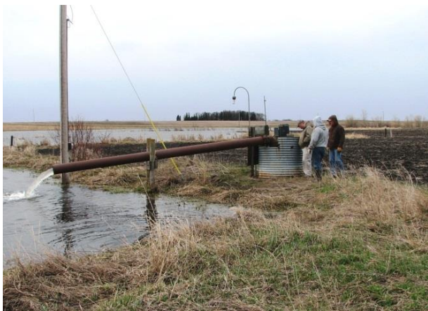
Figure 4. Drainage Lift Station Relocated to Facilitate Restoration of Adjoining Wetland
