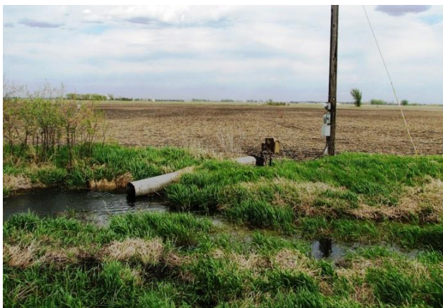
Figure 3. Low Lying Tile Drained Wetland Landscape Aided by Electrically Powered Lift Station
