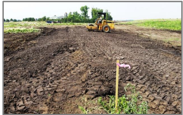
Figure 11. Compaction of Constructed Ditch Plug
