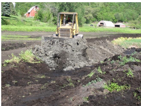
Figure 2. Shallow Ditch Being Filled
