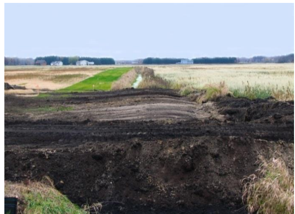
Figure 12. Finished Ditch Plug with Crown in Middle
