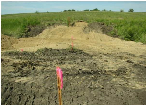
Figure 10. Ditch Plug under Construction
