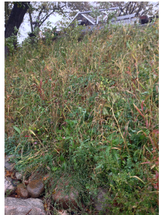
Steep bank stabilized with flowers, grasses and erosion fabric
