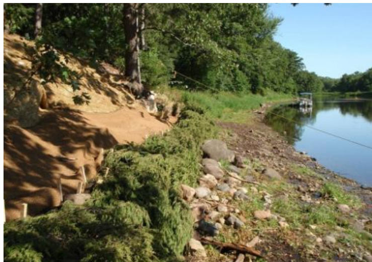
Bank stabilization with cedar revetments and erosion fabric along the St.Croix River
