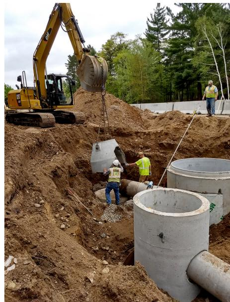
*Crews in late May installed pipes and underground sediment-collectors off Crow Wing County Road 66 just outside Manhattan Beach. The stormwater treatment system will help to preserve Big Trout Lake, the only lake in the county where the Minnesota Department of Natural Resources stocks lake trout. **Photo Credit:** Crow Wing SWCD*
