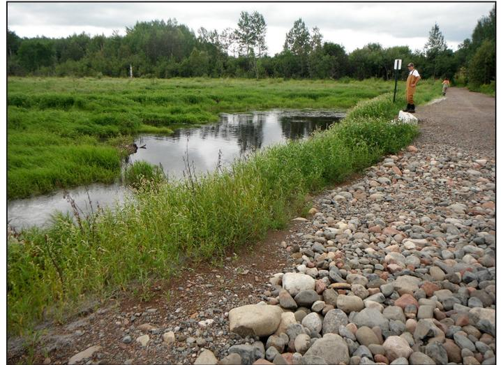
Before-and-after views of a failed culvert and collapsed road spanning Martin Branch, a trout stream that empties into Stoney Brook, illustrate the problem and solution. The culvert was removed and fixed in 2011, and held up well in the 2012 flood. The Fond du Lac Band of Lake Superior Chippewa has since seen the flooded wetland recover and the stream-dwelling macroinvertebrate population improve. **Photo Credits:** Fond du Lac Office of Water Protection
