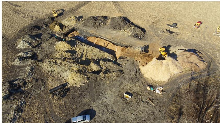
*A drone image depicts a wood-chip bioreactor under construction in Fairbault County.*
