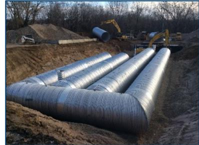
*FROM LEFT: Most of the work to construct a cistern and a series of pipes under the softball field and part of the parking lot at Upper Villa Park in Roseville was completed in late fall 2015. The softball field at Upper Villa Park in Roseville is now irrigated with rainwater collected in an underground cistern. A series of underground pipes perforated with thousands of holes will allow rainwater to seep into the ground. Photo Credits: Capitol Region Watershed District*
