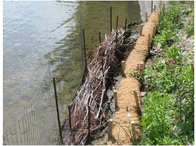
Shoreline restoration using wood mulch, coconut fiber bio-logs, wattles and fencing
