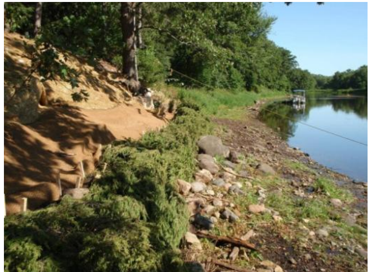
Bank stabilization with cedar revetments and erosion fabric along the St. Croix River
