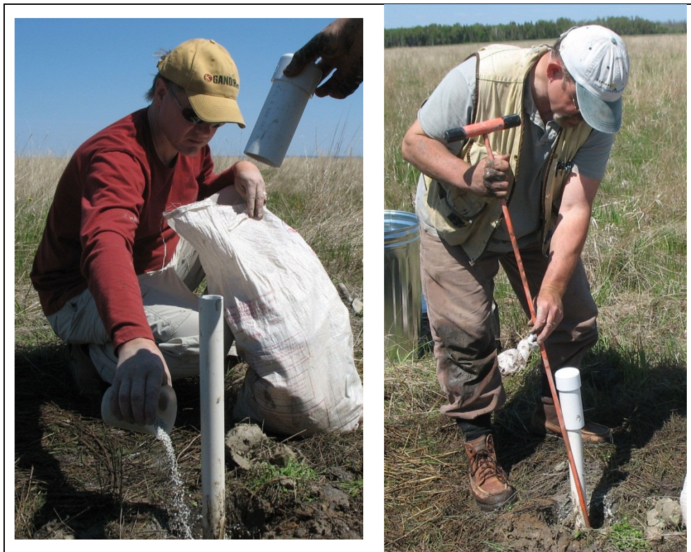
Figure A10: Adding (left) and tamping (right) bentonite.
