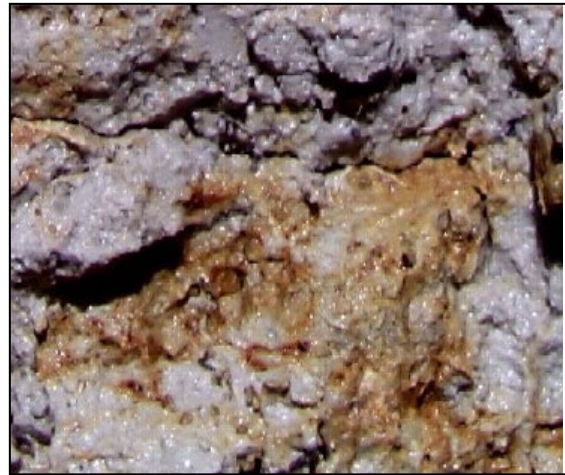
Figure 6: Water glistening on the surface of saturated soil.
