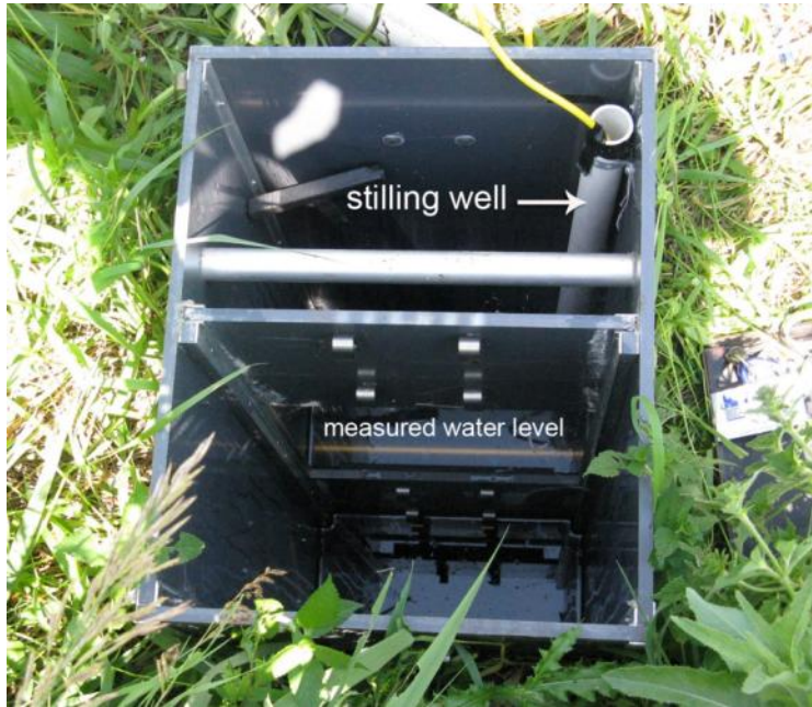
Figure 11: Water control structure with stilling well and data logger.
