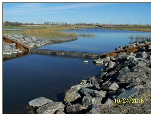
Constructed Weir and Sediment Pond at Peach Creek Diversion Outlet
