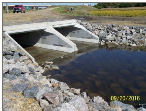
Box Culverts Installed as part of Peach Creek Diversion
