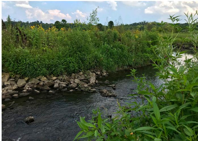
**Top:** The redesigned South Branch of Cascade Creek mimicked the sinuosity, dimension and shape of a stable channel elsewhere in the watershed. **Bottom:** Wetlands eventually will fill with water. Logs and roots will help to create habitat.
