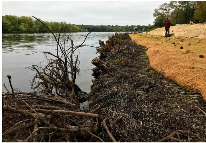
*Jute and coconut fiber-wrapped soil lifts layered with brush "mattresses" of willow, dogwood and alder create toe wood benches along a 600-foot-long stretch of riverbank at Mississippi River County Park. When the shrubs take root, they will help to stabilize the shoreline. Root wads placed on top of logs on the riverbed help to cut the velocity.*
