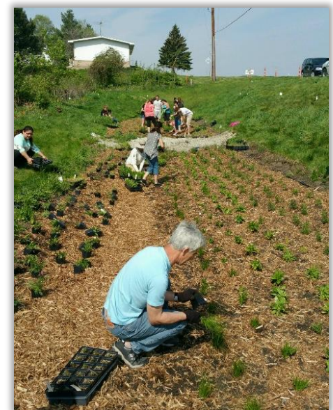
Before work began, top, and volunteers hard at work installing the rain garden, bottom.
