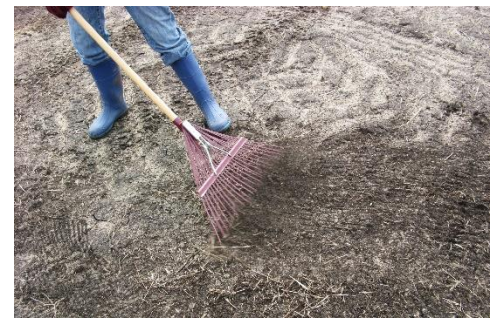
Inter-seeding of a Construction
