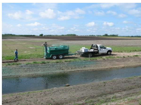
Figure 4. Seeding and Hydro-Mulching a Constructed Ditch Reroute
