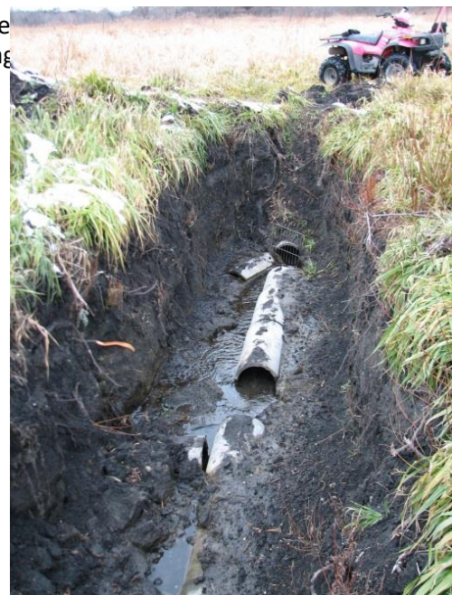
Figure 1. Removing “Blocking” Subsurface Drainage Tile
