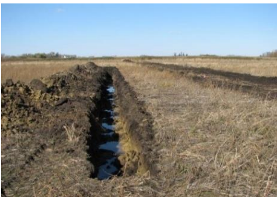
Figure 12. Tile Investigation Trench
