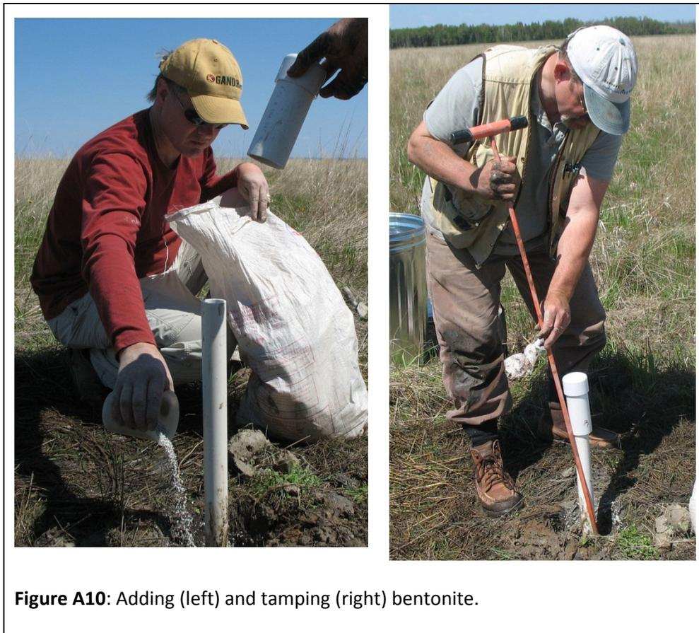
**Figure A10:** Adding (left) and tamping (right) bentonite.
