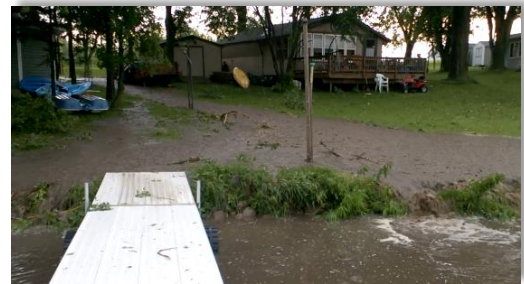
Drainage outlet before
