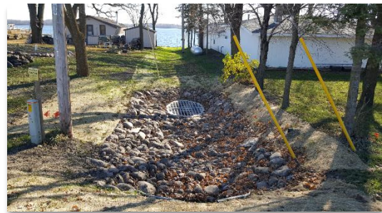
Drainage outlet after
