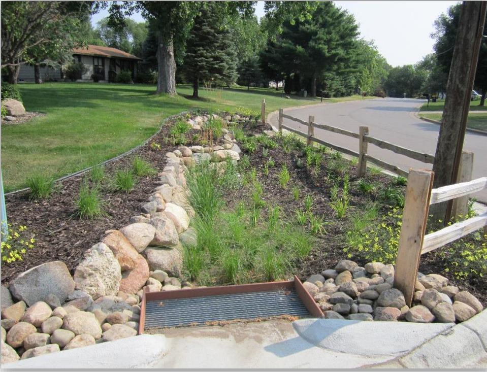
*Left: A curb-cut rain garden and a pretreatment chamber were installed to capture and filter urban stormwater runoff. The plan devised by the Chisago Soil & Water Conservation District leveraged partnerships with three cities, one county, a lake association and rural and urban landowners.*
