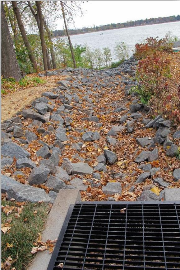
*A pretreatment chamber and a rock-lined chute were installed to capture sediment and stabilize an urban gully as part of a Chisago Lakes Chain of Lakes Watershed project.*
