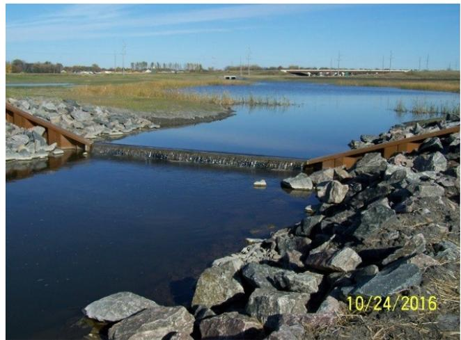
*Sheet pile weir at outlet of Peach Creek diversion sediment pond*
